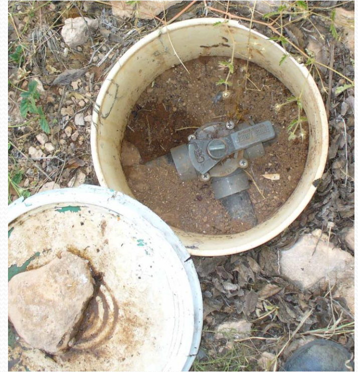
Gray water outlet & diverter valve
