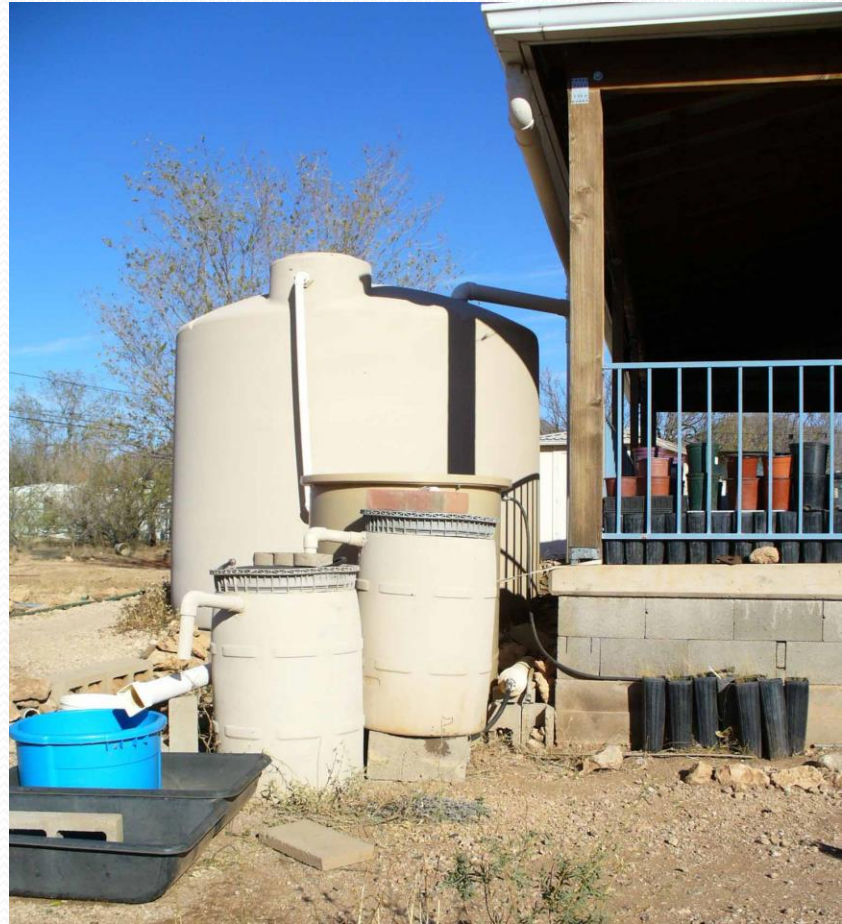
A few of our rainwater storage tanks
